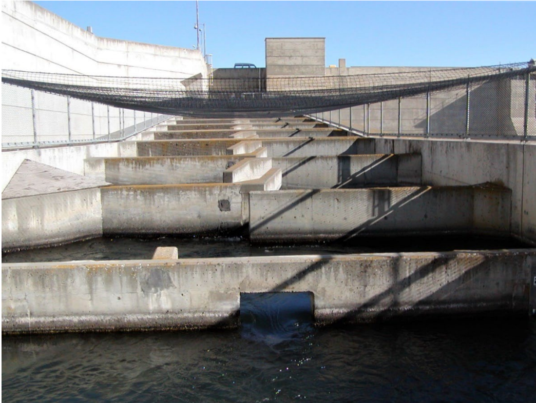
Figure 2-1. John Day North Fish Ladder Serpentine Control Section in 2009 before Modification.
