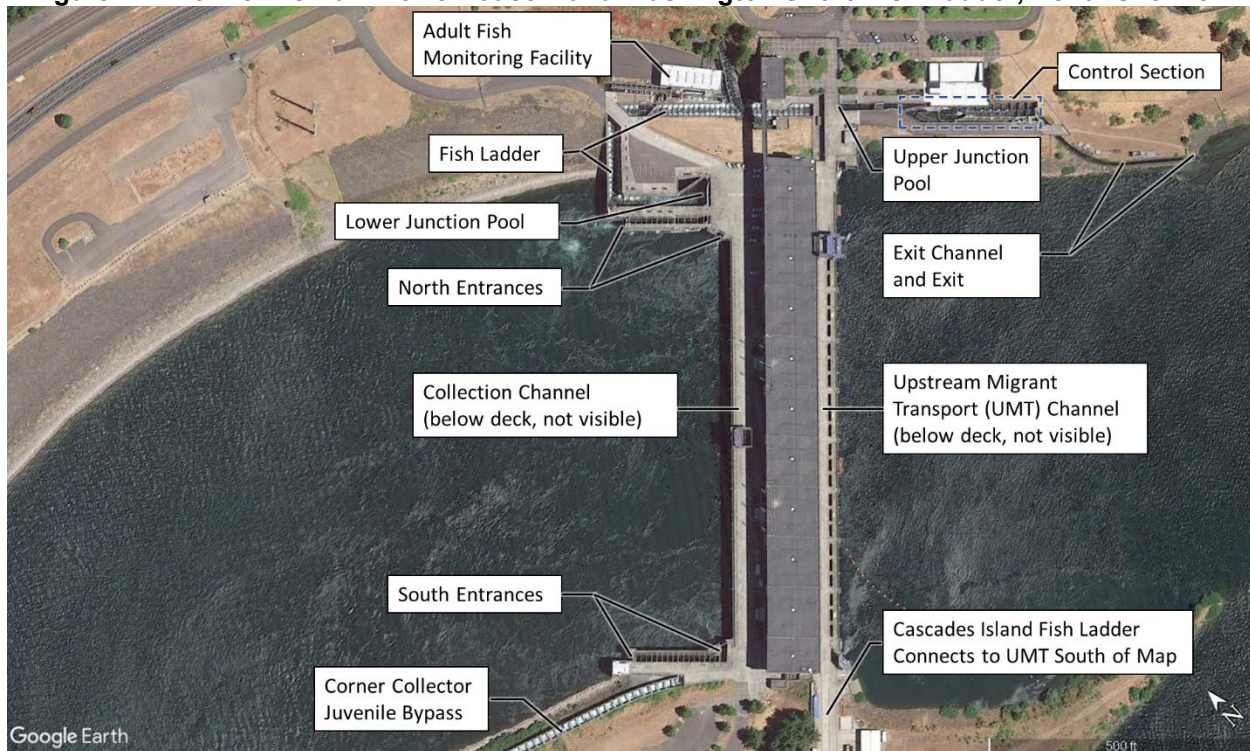
Figure 1-4. Bonneville Dam Powerhouse 2 and Washington Shore Fish Ladder, Aerial Overview
